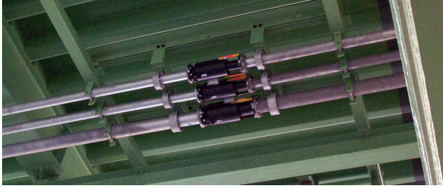
Series 3501 (Axial) Expansion Joint used on a municipal bridge
